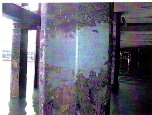
Plate 1. Area of pile cleaned for inspection
